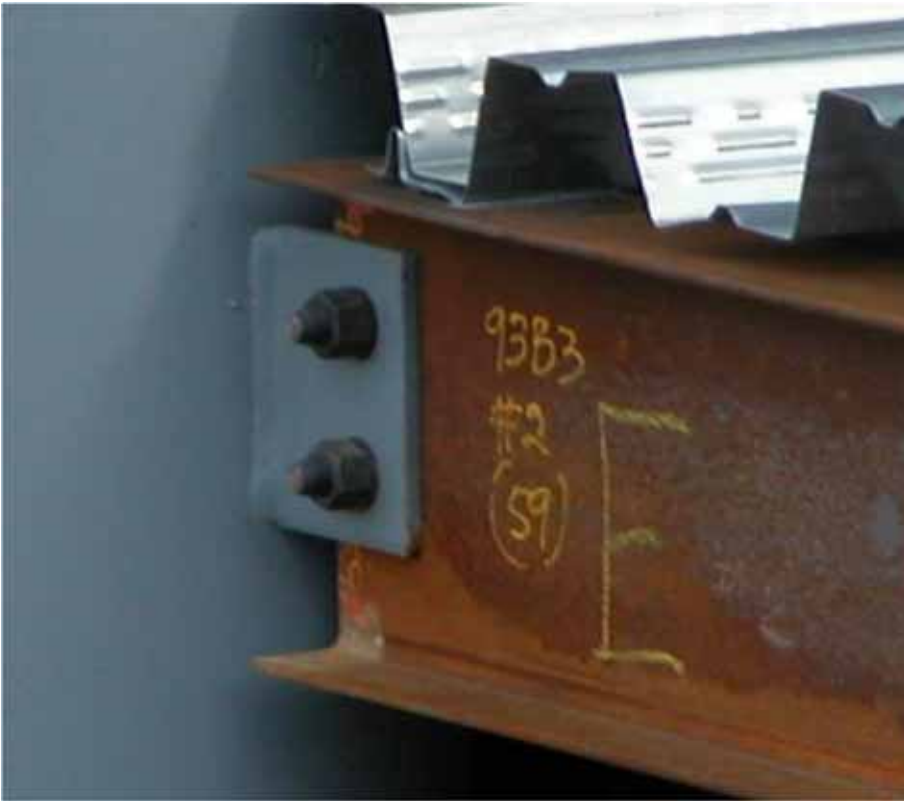
Single Plate Connection (Shear Tab)
