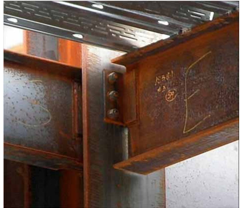
Double Angle Connection
